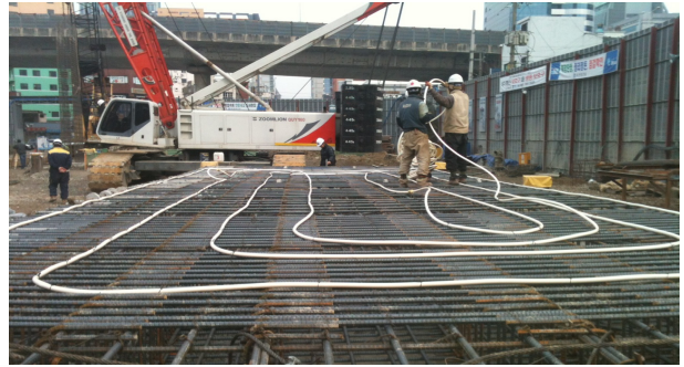
Fig. 2 Construction situation of barrette pile.
