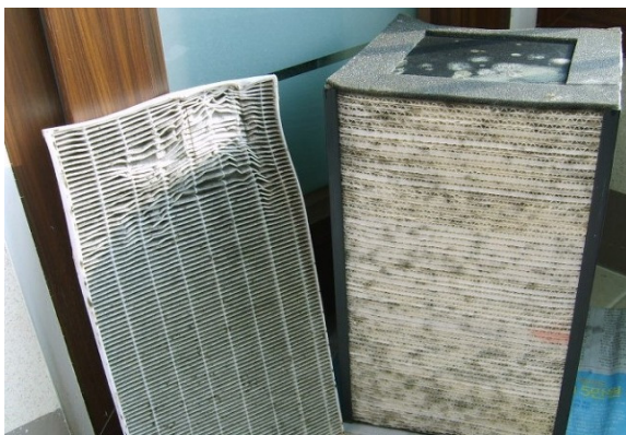
Fig. 2 A photo of a heat exchange core covered with mold.
