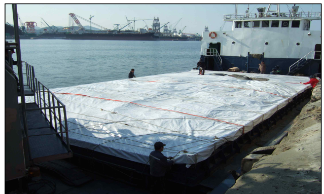
Fig. 2. Photo of covering the hatch.
