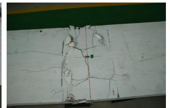
Fig. 14 Failure shape : bottom rebar
