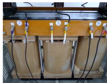
Fig. 4. The arrangement of windings in model transformer.
