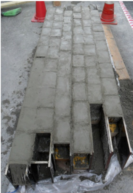
Fig. 4. Specimens after concrete pouring.
