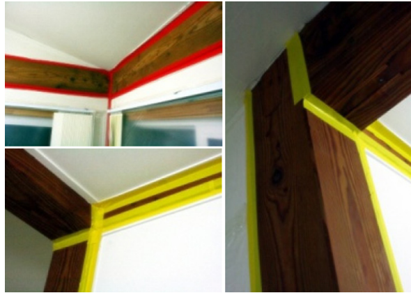
Fig. 6. Taping the gaps between frame and wall.
