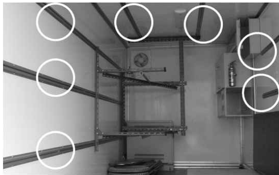
Fig. 13. Supports for installation of additional devices
