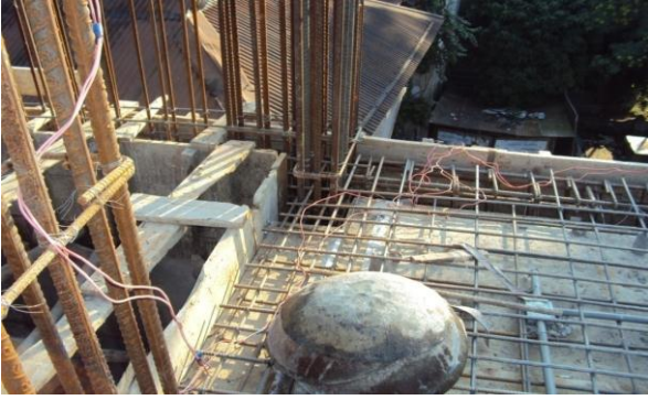
FIGURE XXIII TO KEEP ELECTRIC WIRE AT CASTING PLACE AT KARIM TOWER.
