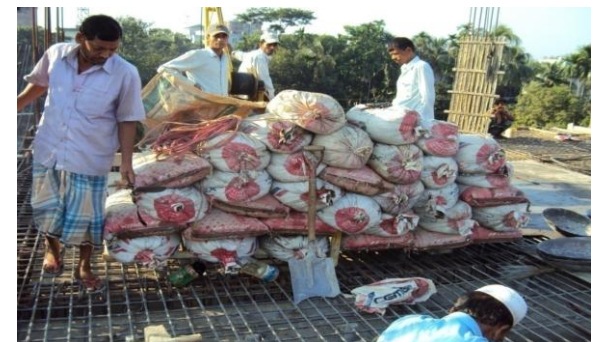
FIGURE XXII BURDEN ON SLAB CASE BEFORE CASTING AT ARK HOMES.
