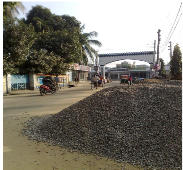
FIGURE XIII MISMANAGEMENT OF CONSTRUCTION MATERIALS AT PUMP TOWER.
