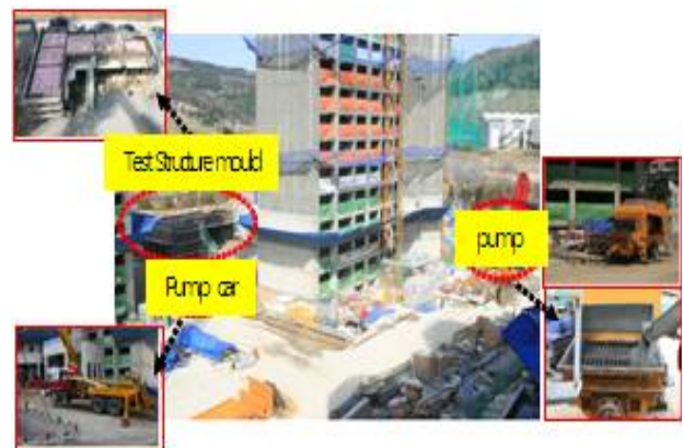
Figure 5. Pumping Placement Plan of Pilot Test
