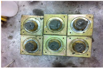
Fig. 2 Spreaded cement mortar
