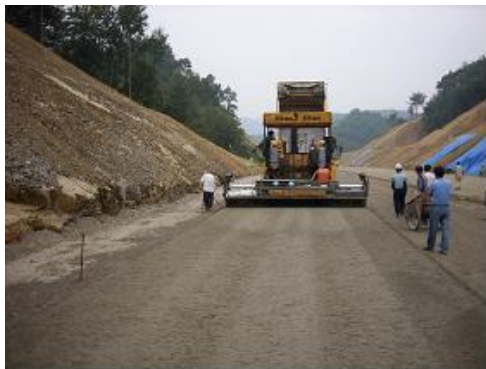
Fig. 4 View of The Test Construction
