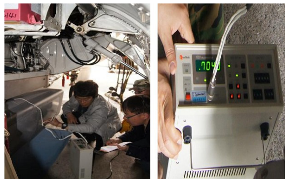
Fig. 10. Ground resistance test
