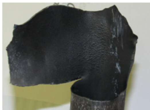
Fig. 1. Damaged Pipe by FAC.
