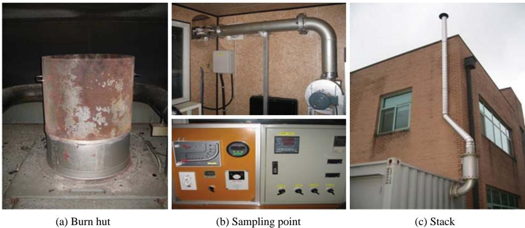
Fig. 2. Diagram of burn hut, sampling point and stack.
