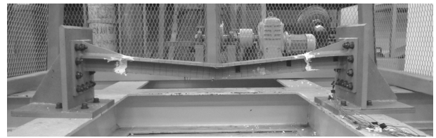
Fig. 6 Overall view of deformed shape
