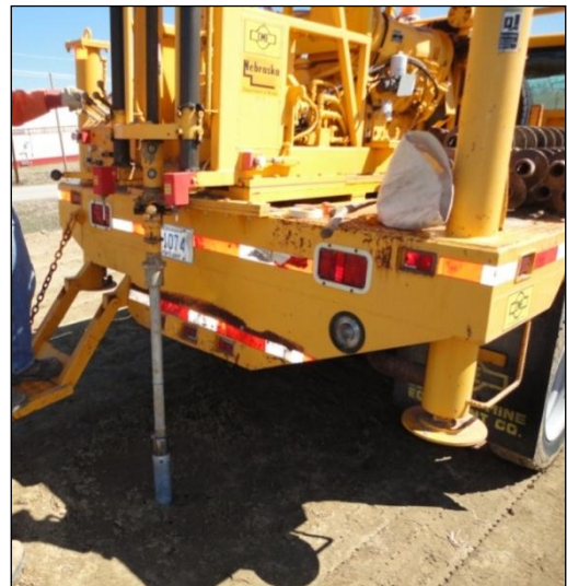
FIGURE I SHELBY TUBE DRIVEN IN THE GROUND
