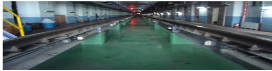
Fig. 1 Depot with iron-beam
