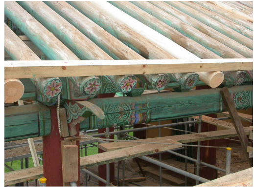
Fig. 3. Jeongjagak, the ceremonial hall under repair (outside).
