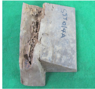
Fig. 7. Cant strip (pyeonggodae) of Jeongjiagak in Seonreung.
