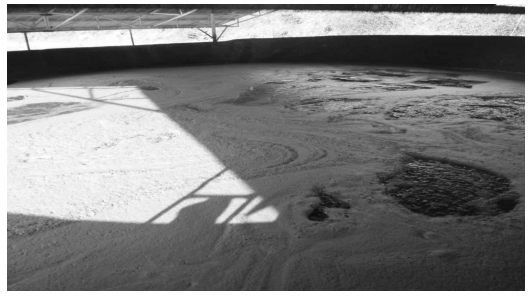
Fig. 20. Slurry mixing with air supply.
