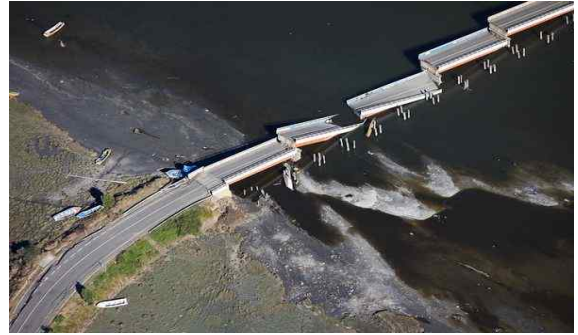
Photo 1. Bridge collapse in Chile.
