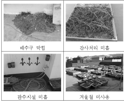
Figure 2. The problem cases of roof garden.
