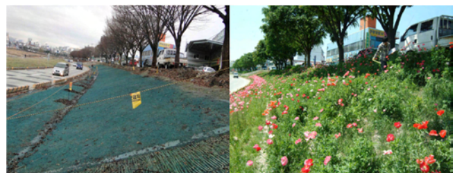
Fig. 9 Seeding completion and environmental monitoring view
