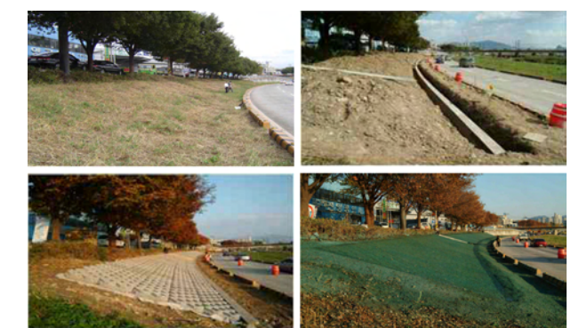
Fig. 2 Field test construction
