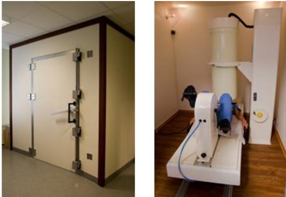
Fig. 6. MCG system installed at AKHH by BMP. Magnetically shielded room (left) and its inside (right).
