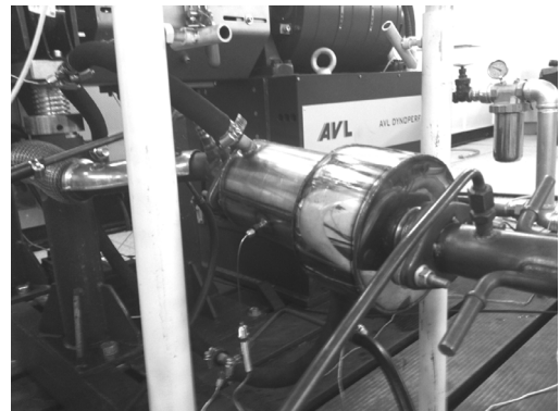
Photo 1 Mounting of exhaust heat recovery device
