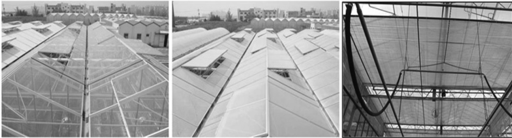
Fig. 1. Shading treatments used in the experiment: Left, the control; middle, a shading agent; and right, internal screen shade.
