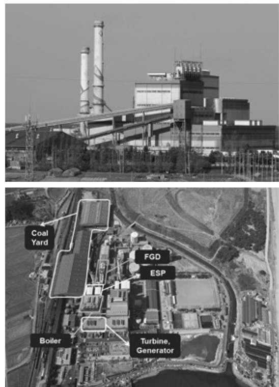
Fig. 1. Birds-eye view of Youngdong Power Station.
