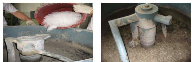
Figure 1. Ice-flake and concrete mixing
