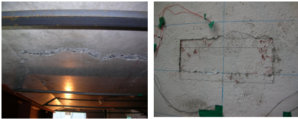
Fig. 6 Typical failure patterns of deck slabs after a test
