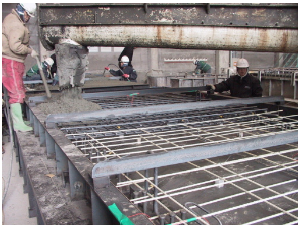
Fig. 3 Manufacturing view of test specimen
