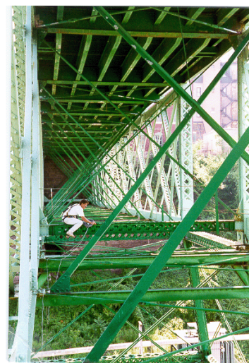
Fig. 3 View of Floor System and Cross Bracing
