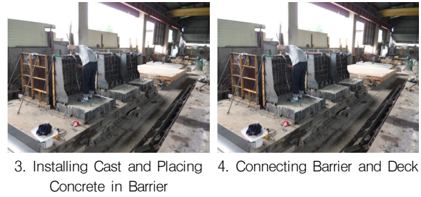
Fig. 6 Procedure of Building Specimen
