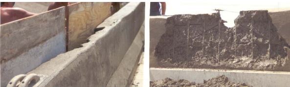
Fig. 3 Barrier Repair
