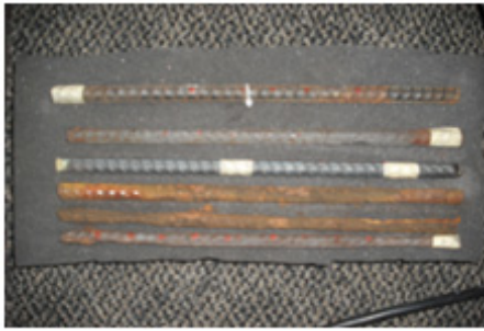
(a) Corrosion in bare rebar
