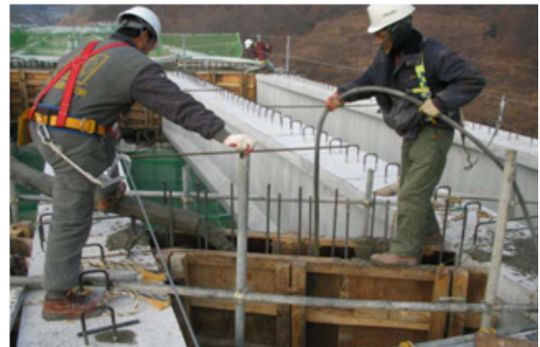
Fig. 1 Placing Diaphragm in Field
