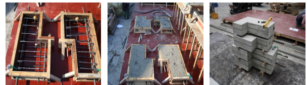
(a) Form and Re-bar (b) Placing Concrete (c) Curing
