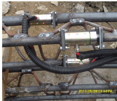
Fig. 7. Load cells installed at the lattice girder.
