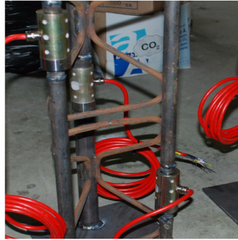
(a) Load cells installed in the lattice girder
