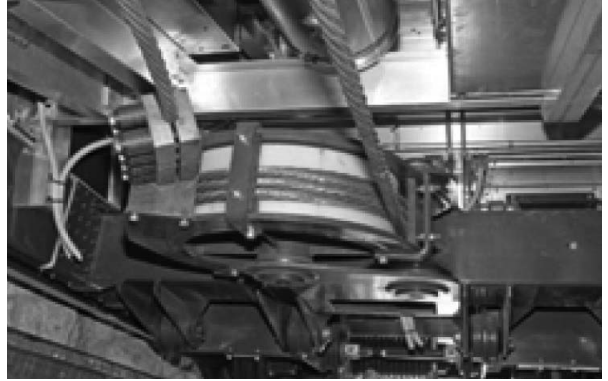
Fig. 6 Winch to drive a car by winding a rope
