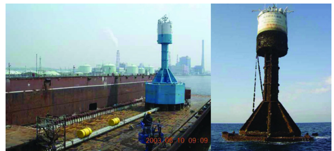
Fig. 2 TAKIUMI developed in Japan (Left : final fabricated structure, Right : installed structure in real sea)
