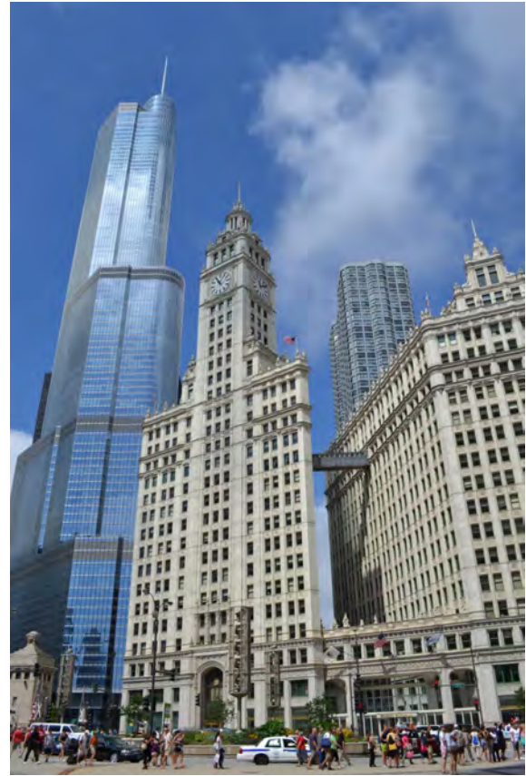
Figure 2. The newly constructed Trump Tower in Chicago. While the design provides a modern-looking tower, yet it respects the historic neighboring Wrigley Building by applying similar modules, horizontal belts, and building top. (Photograph by author)
