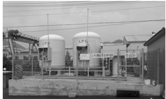
Fig. 2. The shape of gas storage facility.
