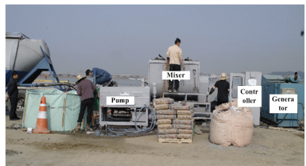
Fig. 4. Mixing system for field test
