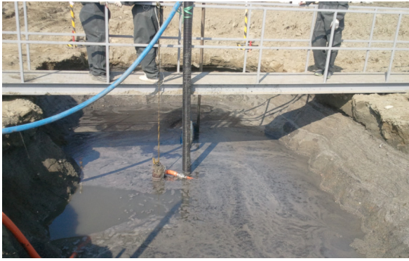
Fig. 5. Placing CLSM
