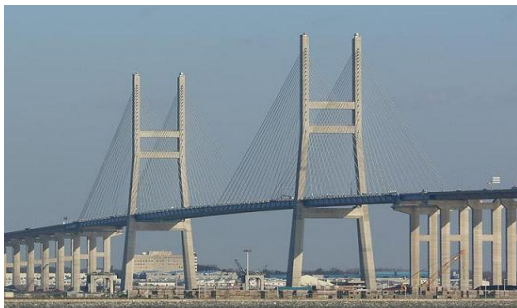
Fig. 16 View of the test bridge
