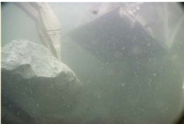
(c) Scene of assembled armor stones
