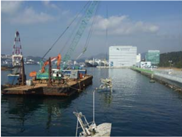
(a) Construction site
