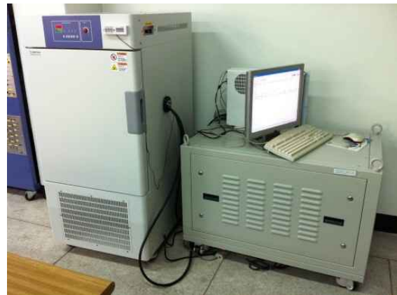
Fig. 6 Temp. Humi. Test Chamber & 5V 100A Battery Cycler
