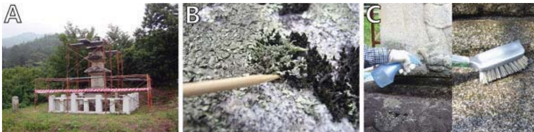
Fig. 8. Scaffolding installation(A) and dry and wet cleaning(B, C)
