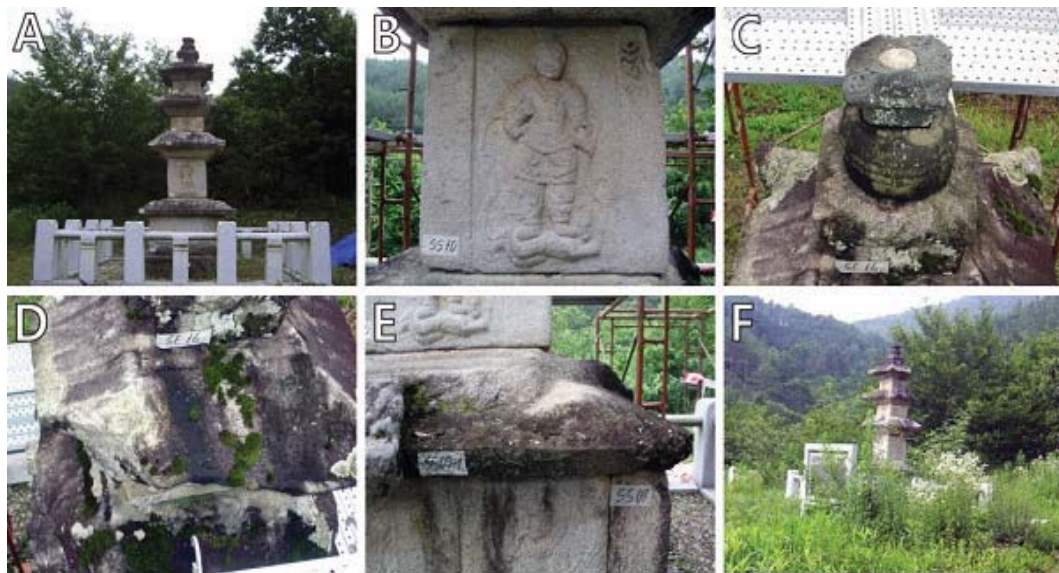
Fig. 1. Site occurrence of the three-storied stone pagoda in Seungansaji temple site. (A) Panoramic view (B) First story (C) The pole hole on the top (D) Biological colonization on roof stones (E) Cement mortar of the basement stone (F) Forested surrounding environment
