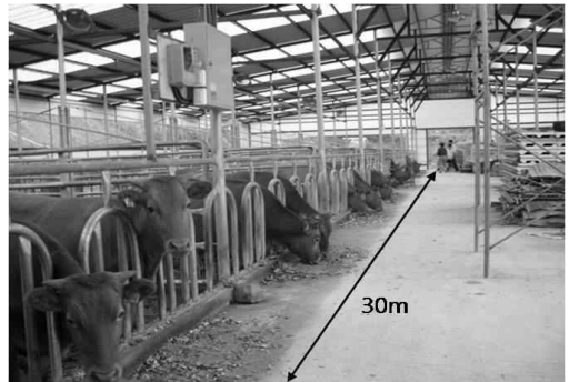
Fig. 14. Internal length of cattle shed.
