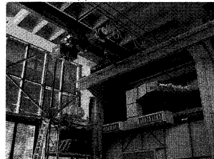
(b) Hoist crane
