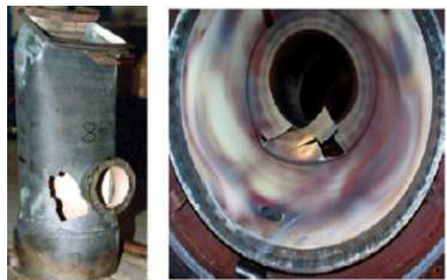
Fig. 2 Combustors damaged from combustion instabilities (Ref. (2))
