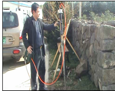
Figure 3. Working posture after using the Pile Driver
