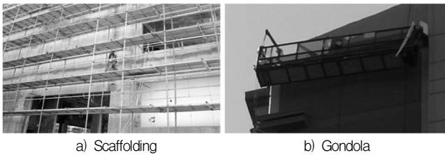
Figure 5. Temporary equipment for exterior insulation and finishing works
