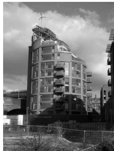
(c) The Green Building, Macintosh Village, Manchester
